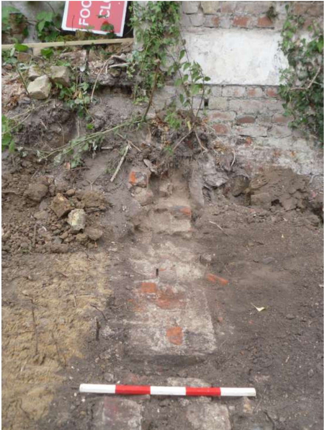
Plate 6, View of modern foundations to the east of the site
