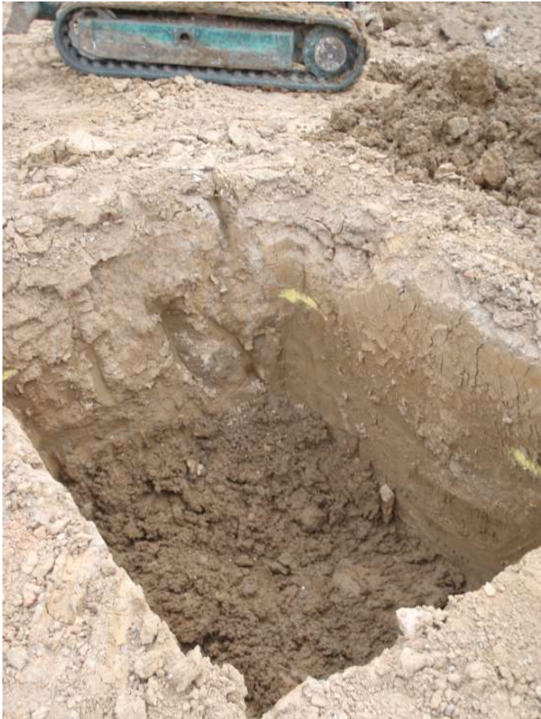
Plate 3. View of drain excavation
