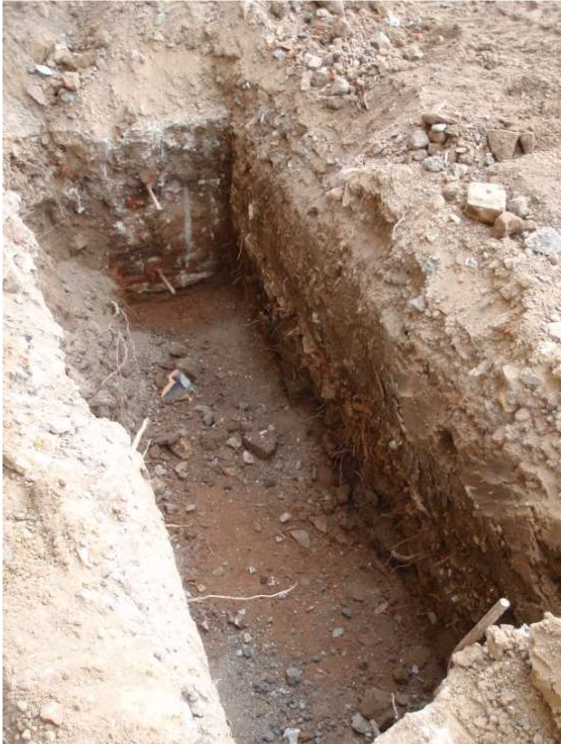
Plate 5, View of foundation trenches to the front of the site (east side)
