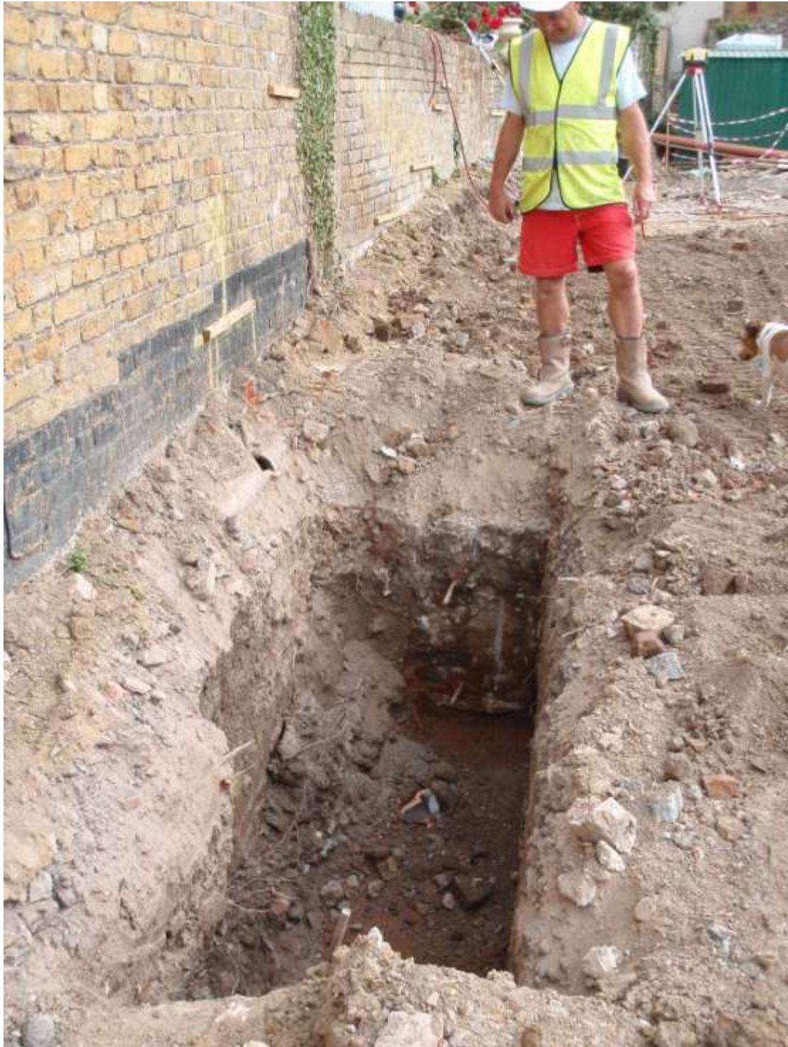
Plate 4. View of foundation excavation at the front of the site (west side)
